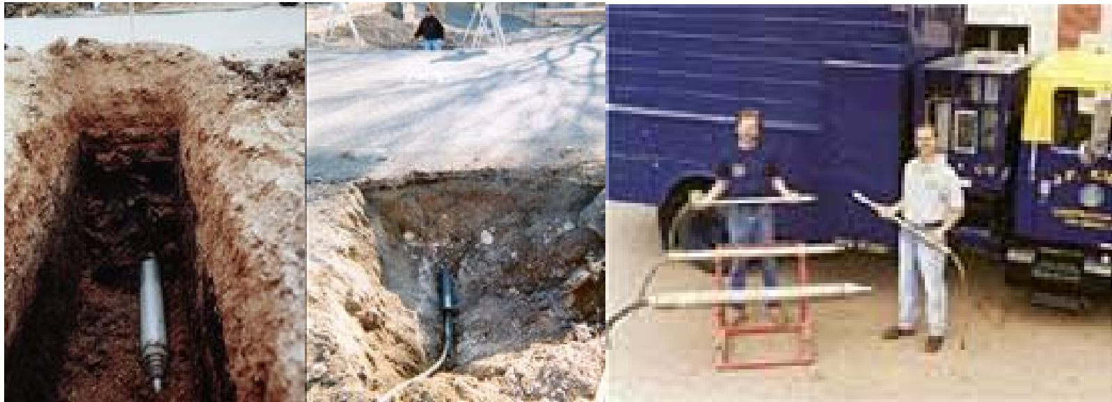
Piercing Tools, pulling a utility behind the piercing head
